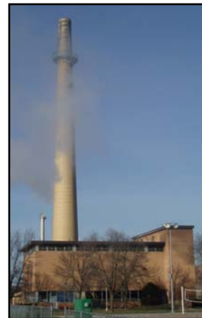
UW-Eau Claire's Coal-fired Power Plant
