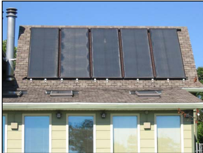
Eau Claire home utilizing both passive and active solar energy
